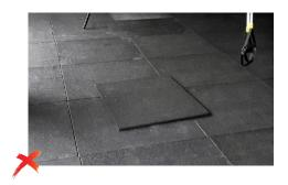
7) If some seams are gapping it is possible to hold them together temporarily with blue painters tape. Tape MUST be removed after adhesive has developed a firm set which is approximately 2-3 hours. Allowing tape to remain longer than 2-3 hours or using aggressive tapes may result in adhesive residue.
