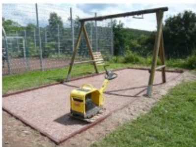
Crushed stones bed stable compacted
