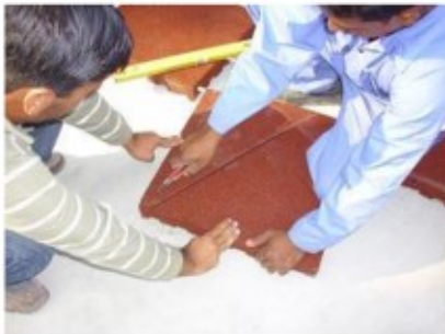
- Cutting with cutter knife
