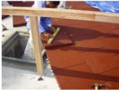
Cutting slabs with a stable cutter knife - Measure and mark cutting edge
