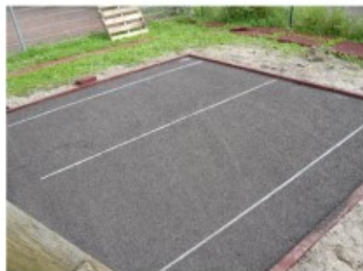
Levelling crushed sand/stone chipping
